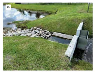
Water control structure between ponds H & K The water control structure is in good condition and free of excess vegetation that could slow drainage.
